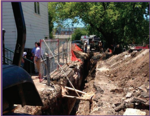
An updated view of the construction site, showing storm drainage lines being installed.
