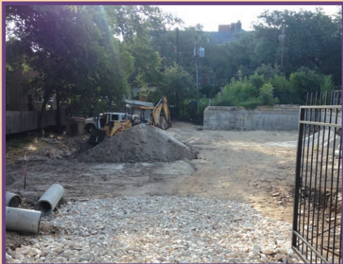
An updated view of the construction site, showing storm drainage lines being installed.
